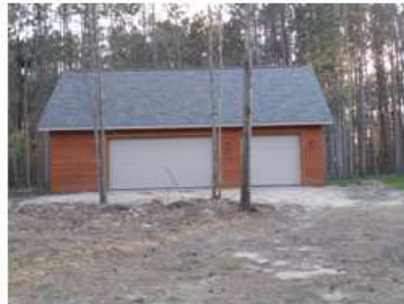
Michaywe Garage with post and beam construction
