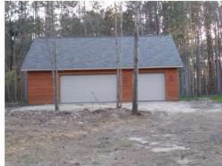
Michaywe Garage with post and beam construction
